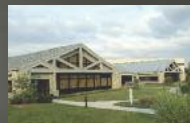
The WL Gore manufacturing plant
